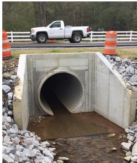
Figure 8.17: Example Drainage Structure
