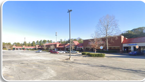
2. Tri County Station
